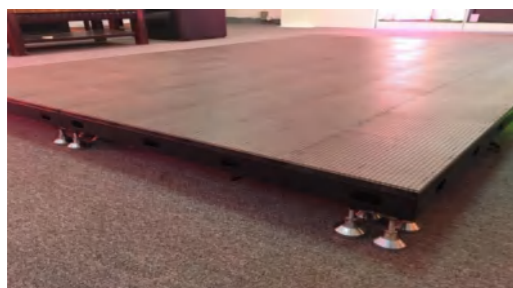
地托安装 Ground support installation
